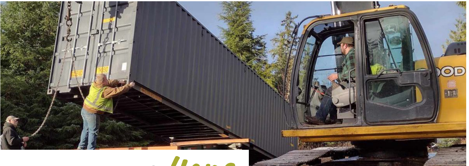
The POWIFB shipping container is relocated to its new site.
